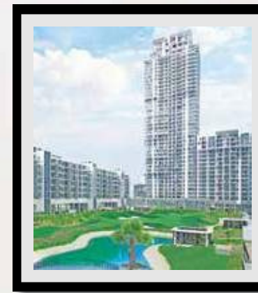
M3M golfstate Fairway GOLF COURSE ROAD EXTENSION SECTOR-65, GURUGRAM
